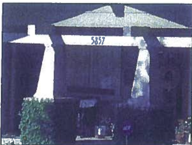
Tapered, Square Piers: Square-shaped posts that connect an overhanging structure to a foundation and have tapered ends.
