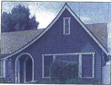
Flared Eaves: A roof edge that curves up and outward in a similar fashion to the curve of a bell.
