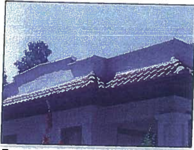
Parapet: A wall projection that rises above the adjacent wall or roof. It can be solid or pierced.
