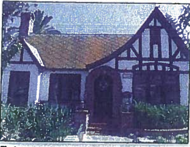
False Half-timbering: Purely decorative timber framework that is filled in with plaster.
