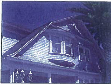
Gambrel Roof: Consists of a short, shallow pair of slopes above another pair of slopes that are steep and curved in a similar fashion to the flare of a bell.
