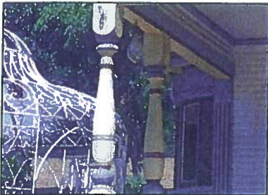
Spindle work: A tapered, decorative wooden post that has been turned on a lathe; often featured on porches.
