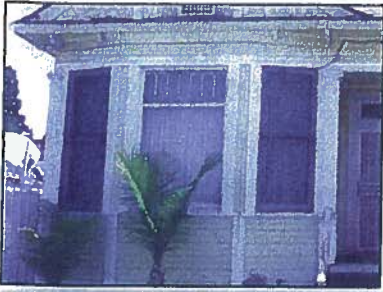
Bay window: A popped out section of the main wall of a house that has a foundation, a roof, and windows.
