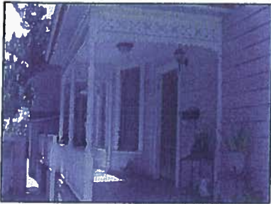
Decorative Millwork: Wood work with ornamental features that is produced in a mill.
