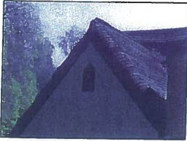
Rolled Eaves: A roof edge that curls downward and in toward the wall.
