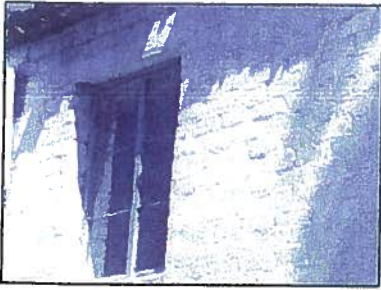
Steel sash casement windows: A window enclosed in steel casing that swings in or out from the wall.
