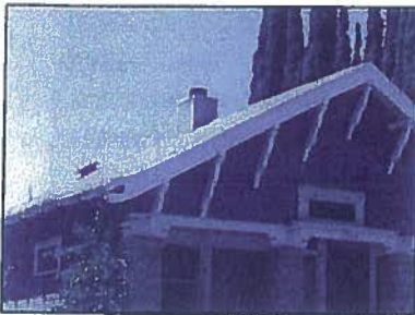
Exposed Rafter Tails: The rafter ends which project beyond the eaves.
