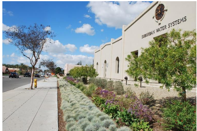
A public water utility company in Whittier
