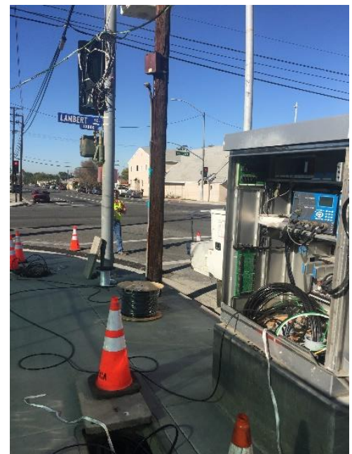
Traffic signal maintenance along Lambert Road
