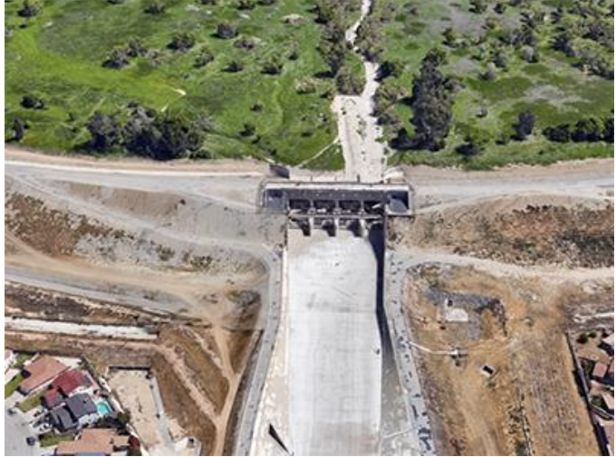
Whittier Narrows Dam Courtesy of the US Army Corps of Engineers
