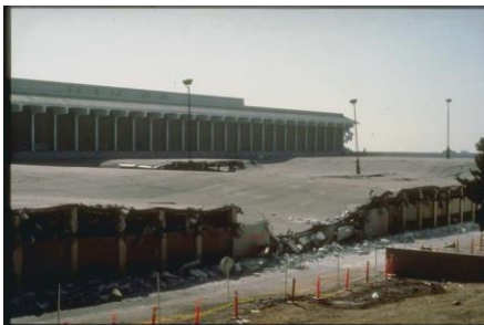
Photo: Partial collapse of parking garage and store (Source: NOAA)
