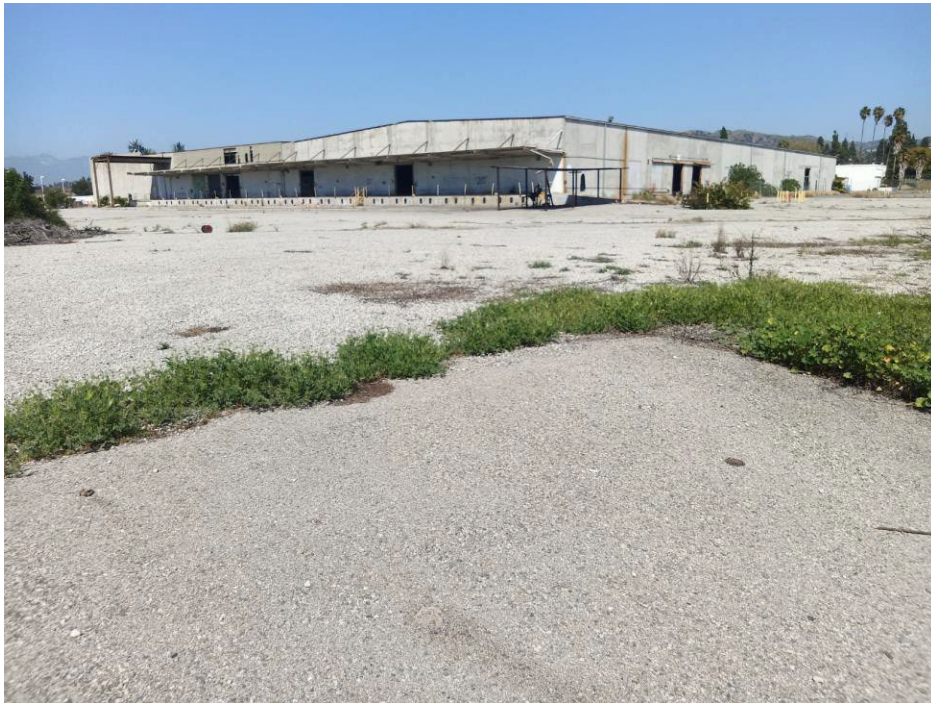
Photograph 11: View looking northeast at the rear or west elevation of the mid-1950s warehouse.
