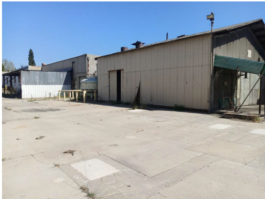
Photograph 16: Close-up of the sheds on the north elevation of the warehouse complex.
