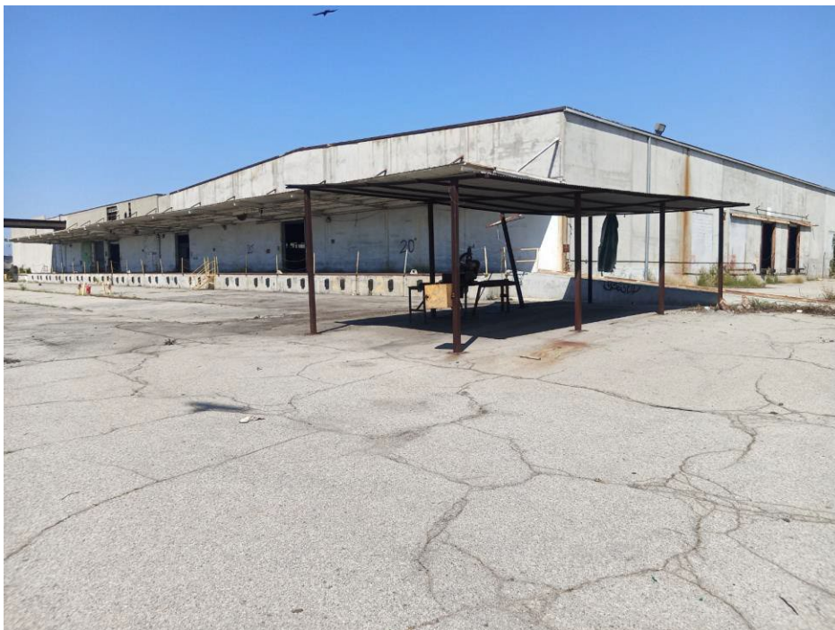
Photograph 12: Close-up of the rear of the mid-1950s warehouse.
