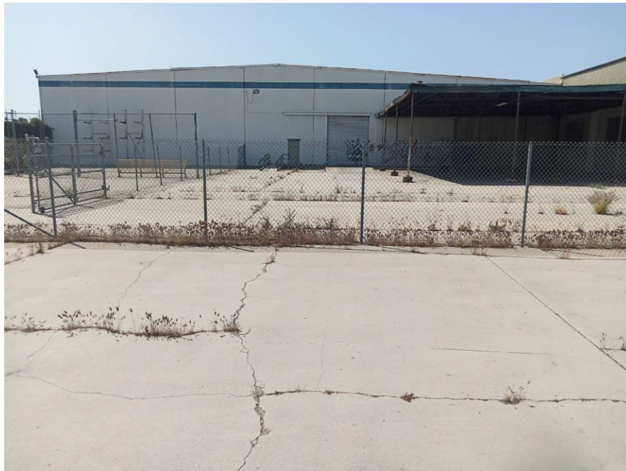
Photograph 8: View looking southwest at the east elevation of the second, mid-1950s warehouse.
