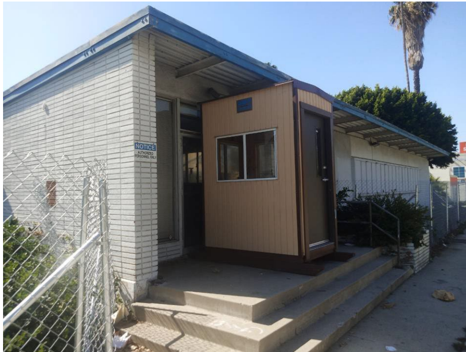
Photograph 19: View looking north at the south corner of the original Ekco Products Company office.
