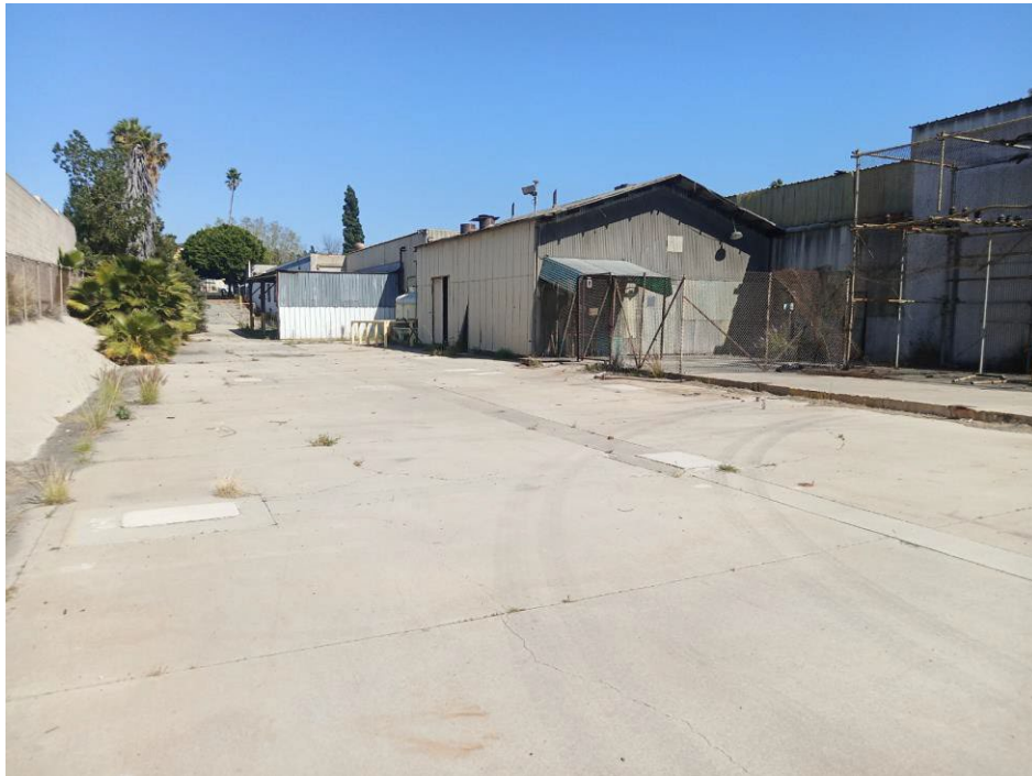
Photograph 15: View looking east at the north elevation depicting the various warehouses and sheds used in the former Ekco Products Company operations during the late-1950s.
