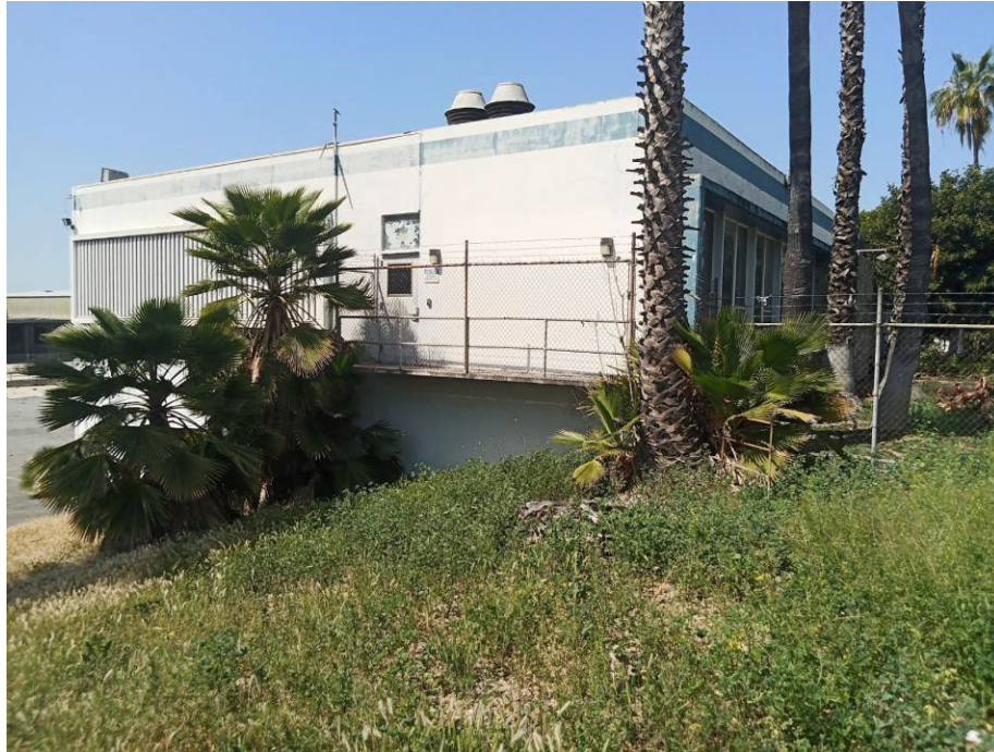
Photograph 3: View looking north at the south elevation of the first Ekco office.
