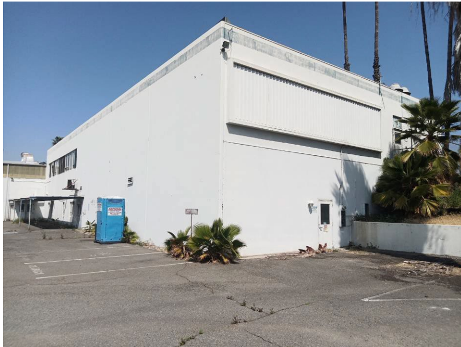
Photograph 4: View looking northeast from the parking level towards the rear and side elevation of the first Ekco Products Company office.
