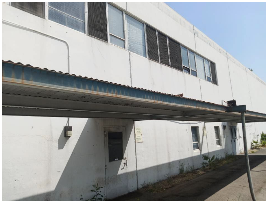
Photograph 6: Another view of the rear of the office looking south.
