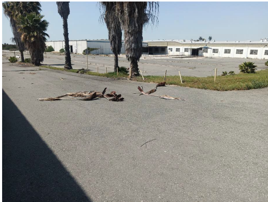
Photograph 2: View looking northwest at the now vacant sprawling warehouses built between 1950 and 1967.
