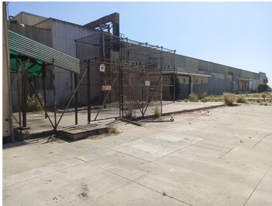
Photograph 14: View looking at the north elevation of the late-1950s warehouse.
