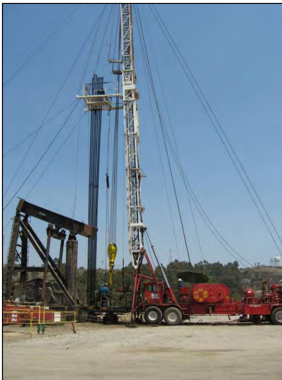
Maintenance Workover Rig
