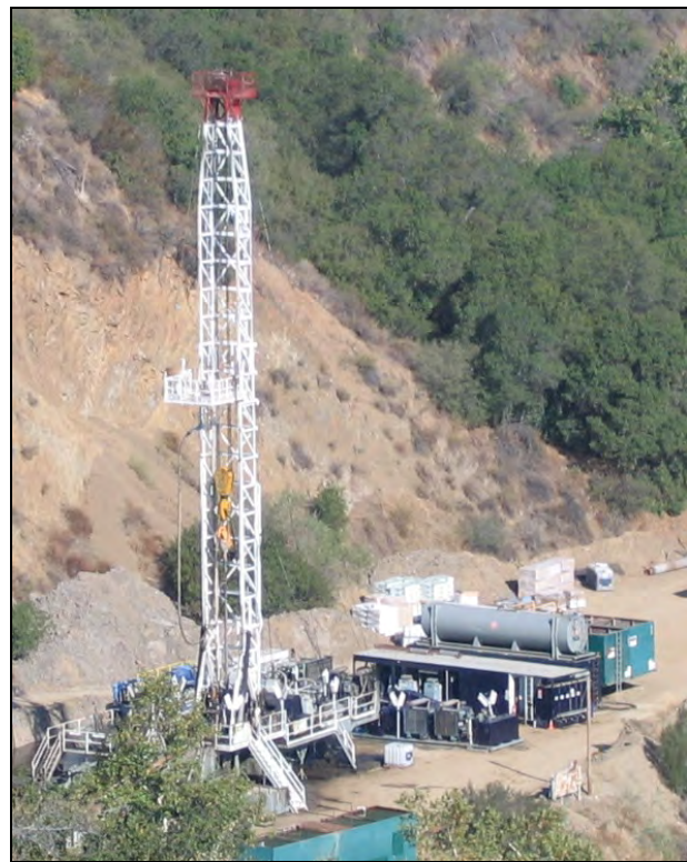
Well Drilling Rig
