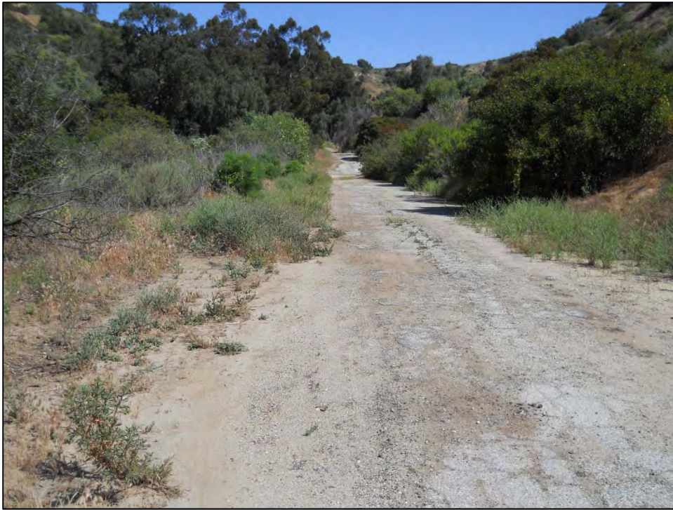
Figure 5.2 Paved access road.
