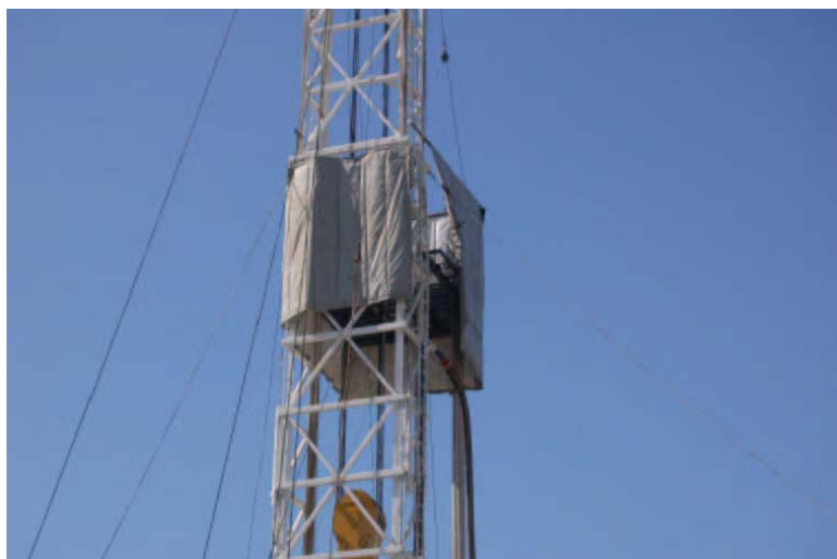
Sound Barrier Around Mast Boards
