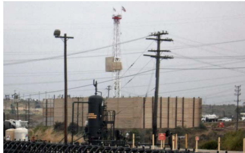
30-Foot Sound Barrier Wall Around Drilling Area
