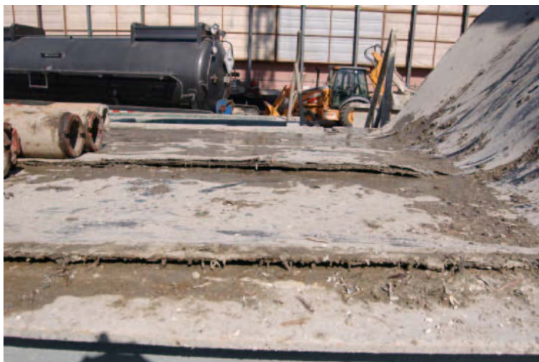
Pads on the Pipe Storage Area and the V-door
