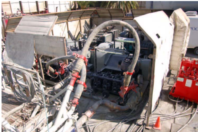
Sound Barriers Around Mud Works and Pumps
