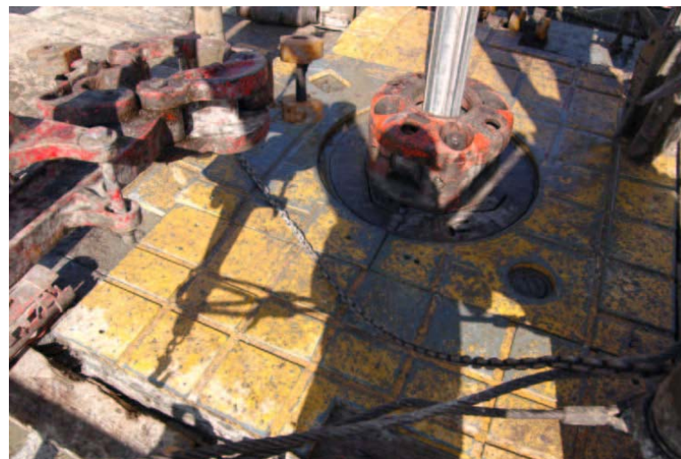
Pads on the Drill Floor
