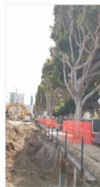
500 Broadway: Collaboration with applicant & 3 rd party arborists opening an exploratory trench to review and mitigate conflicting roots for steel-beam installation prior to excavation & shoring. GC waters trees monthly & provides plant health care treatments for sustained tree health during demo and construction. Trees were methodically pruned for property line clearance & tower crane installation of 8-story structure to be developed to the property line.
