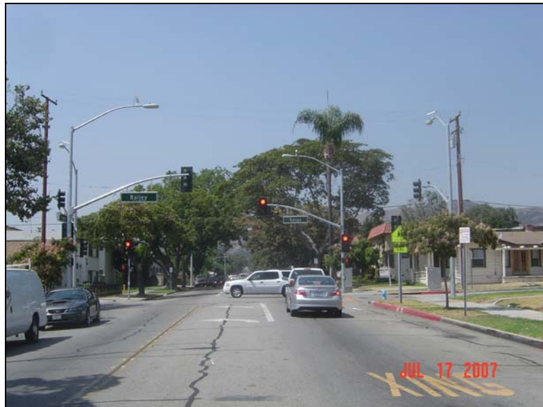
New Pickering Avenue at Bailey Street Traffic Signal
