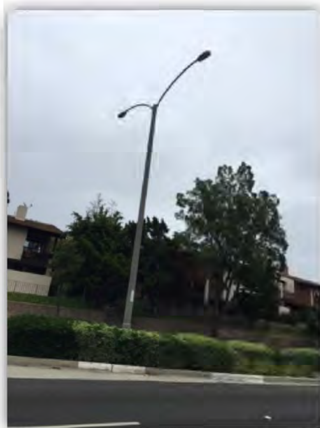
Example of LED energy efficient street light
