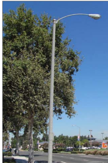
Sorensen Avenue Frontage Lighting
