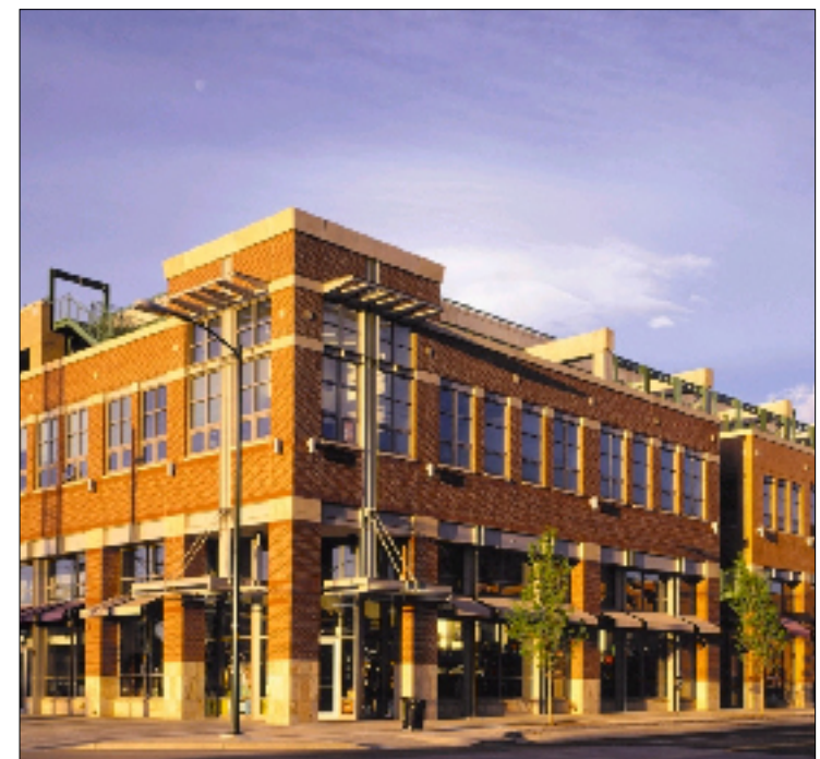
Below: A Park Once structure with retail on the first floor and an architecture that is sensitive in scale and materials to the surrounding urban fabric.
