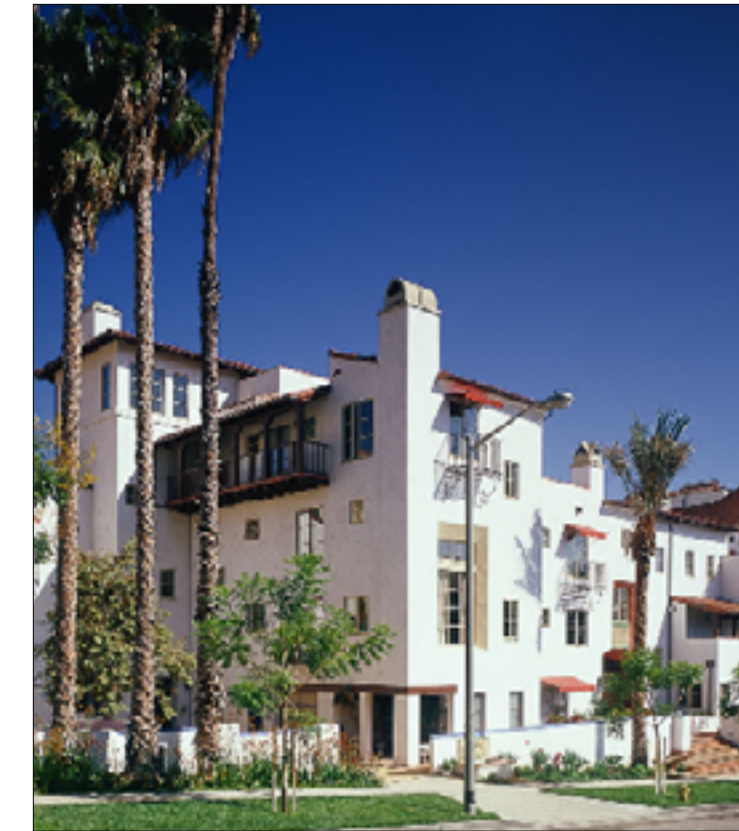
Above: Courtyard housing of about 20 - 35 units per acre, designed with live/work spaces around a series of courtyards and gardens within an urban context.
