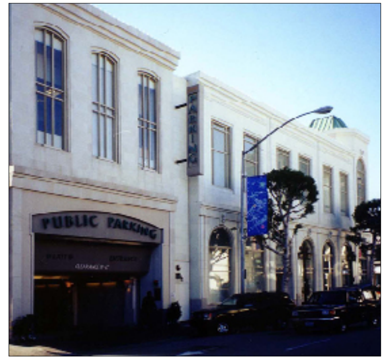
Above: Parking structure integrated with retail and commercial uses in a Liner building type with pedestrian scale facades and clearly marked parking signage and entrance.
