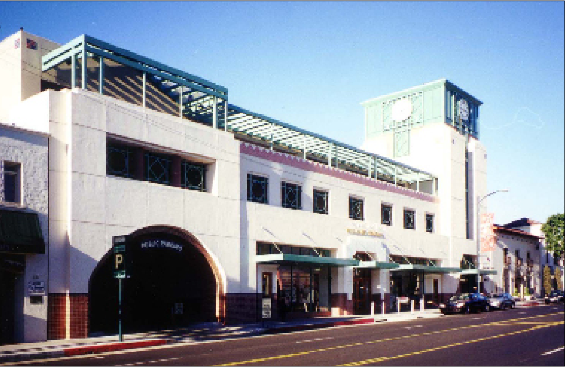
Below: The heart of the Park Once system lies in the parking structures embedded within Liner building types, as shown below, and further described in Chapter 4. From an urban design perspective, retail or commercial uses on the building frontage combined with context-sensitive architecture make such structures 'good neighbors'.
