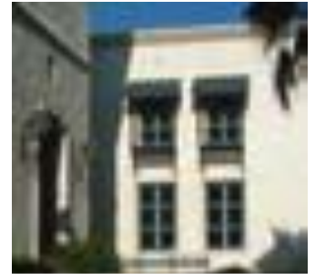
Decorative treatment include awnings and window grilles
