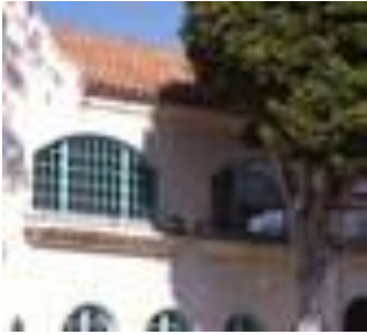
Inset windows with metal framing and grilles on a Spanish Colonial building
