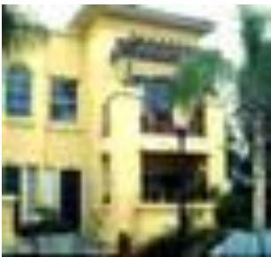
Stucco should create the appearance of thick wall with deeply inset openings
