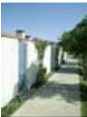
Design elements such as piers should be used to break-up long screening walls
