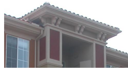
Decorative brackets under eaves
