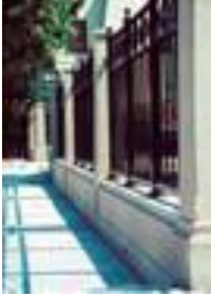
Combine thick and thin structural elements, like thick stucco walls in combination with thin wrought iron
