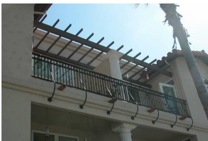
Scuppers are designed and placed as architectural elements
