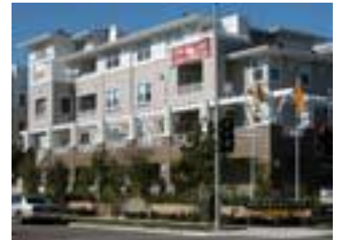
Expanding housing on the Boulevard
