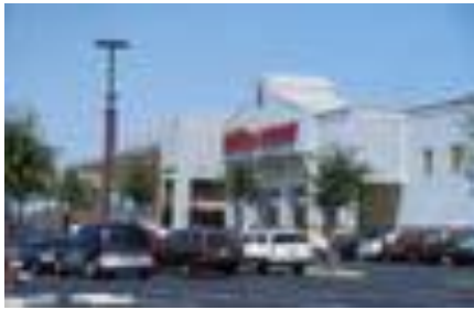
Retail entrances should be highly visible
