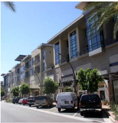
Second floor residential component utilizes same materials as first floor commercial uses, but smaller scale glazing is used
