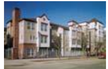
Individual roof forms break up larger buildings
