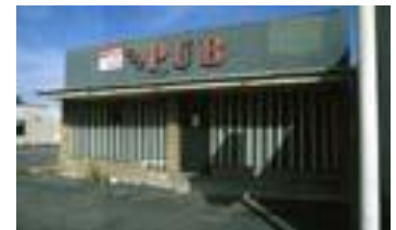
Vacant building on the corridor
