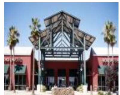
Use building architecture as signage, instead of pole signs
