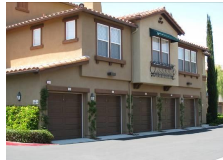
Raised-panel, recessed garage doors with trim add to articulated façade
