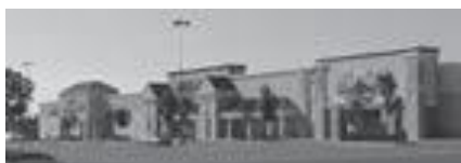
Roof variation on big-box retail
